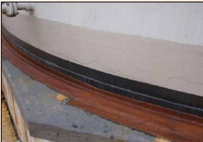
Protection of high temperature tank chime
