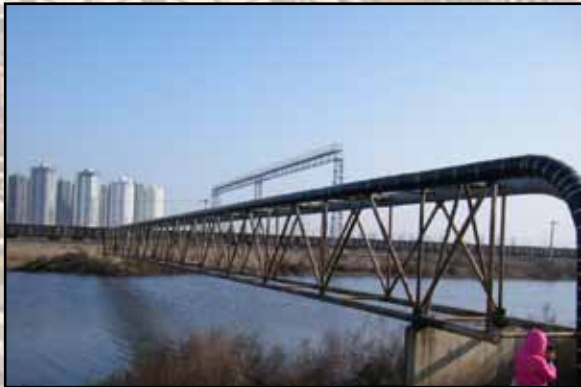
Insulated pipeline across bridge
