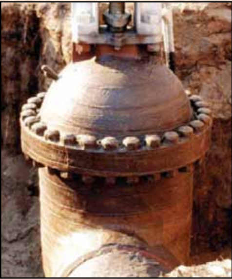
Protection of large valve
