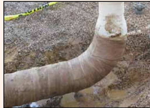
High Temperature Wax-Tape HT-3000 with MC Outerwrap
