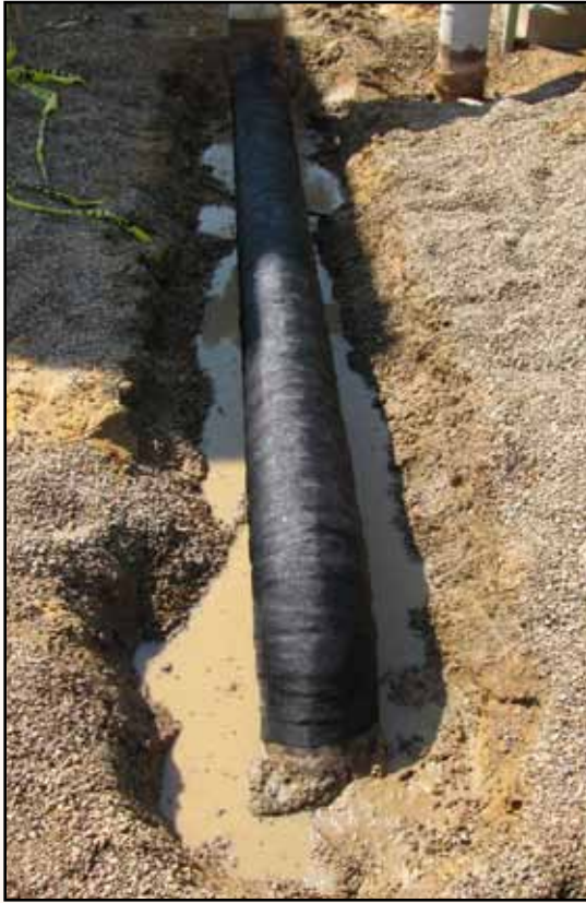
High Temperature Wax-Tape HT-3000 with MC Outerwrap
