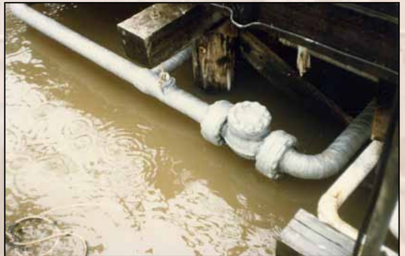
Highly corrosive environments
