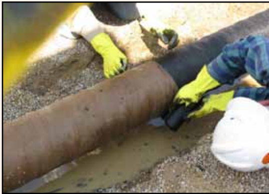
High Temperature Wax-Tape HT-3000 with MC Outerwrap
