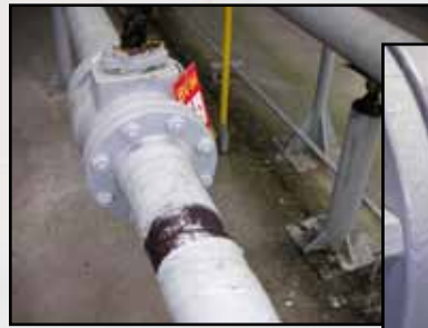
Wax-Tape cut for inspection and repair
