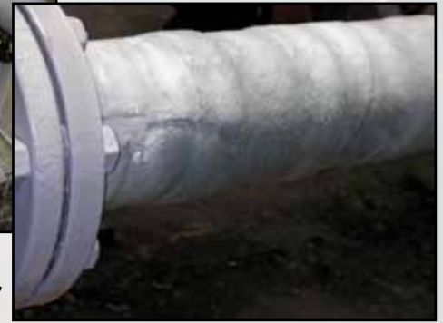
Wax-Tape cut for inspection and repair
