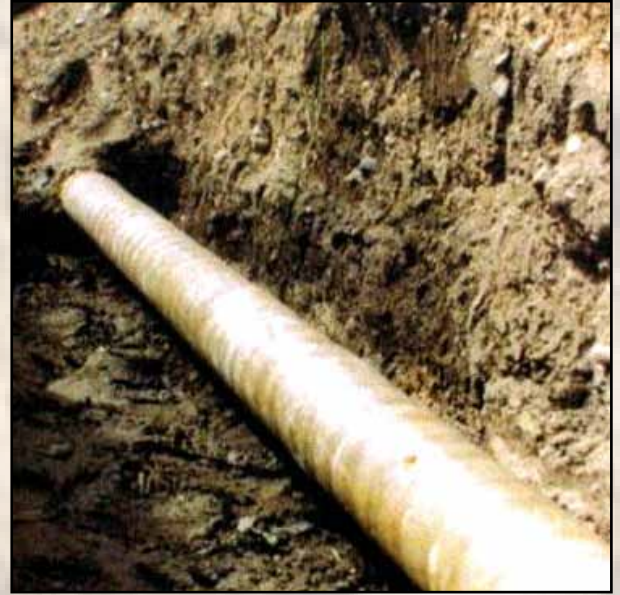
Below ground pipeline can be backfilled immediately
