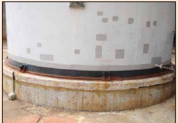
Protection of high temperature tank chime
