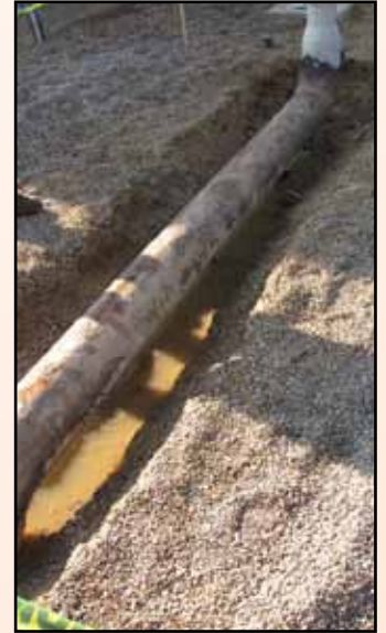
Minimal surface preparation (SSPC SP2)
